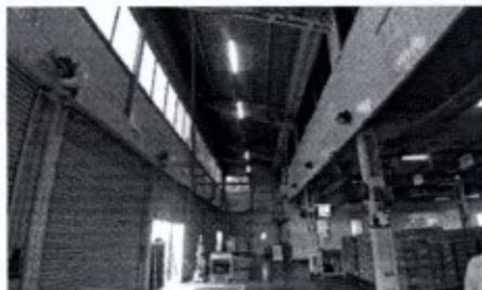
C Building Input Dock
