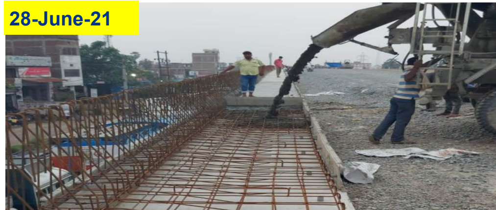
Friction Slab Casting at Km- 208+850 RHS
