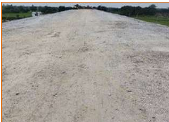
GSB Top Layer completed @ km 157+600 to km 157+790 LHS
