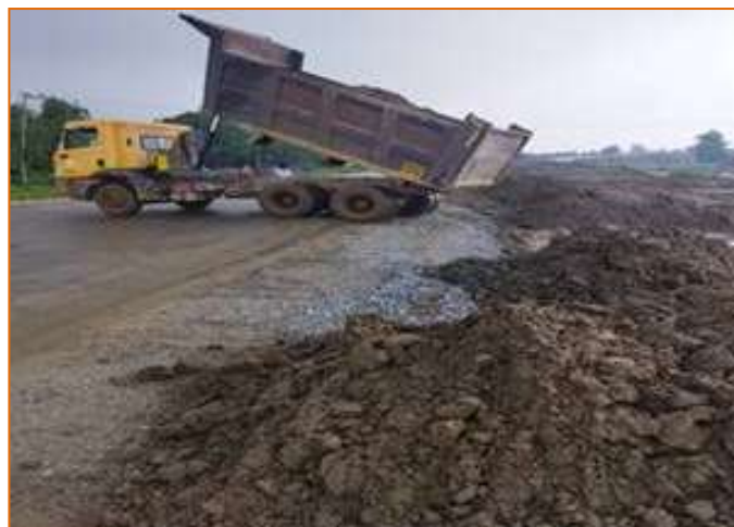
Dumping of soil in progress for Shoulder preparation @ km 158+500 LHS
