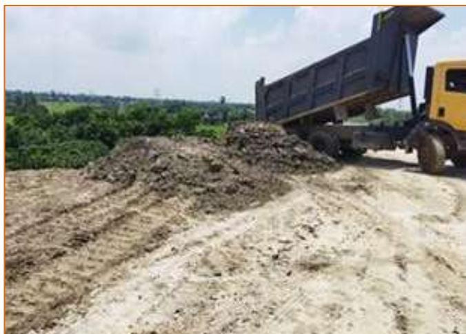
Dumping of soil for Embankment Top layer @ km 157+910 to km 158+050 LHS in progress
