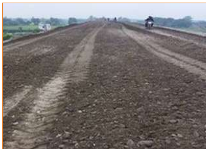
WMM 1 st layer in progress @ km 157+500 to km 157+790 LHS
