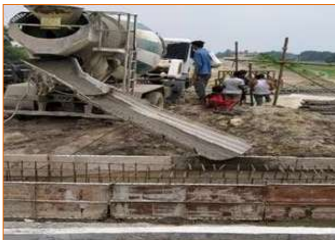
Casting of Raft of Pedestal @ km 157+175 in progress
