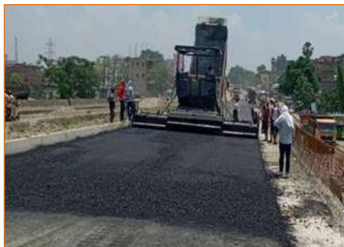
Laying of DBM 1 st layer in progress @ km 207+980 RHS
