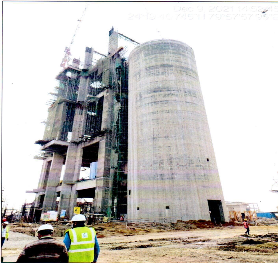
6 Stage Preheater Building and Fly ash Silo
