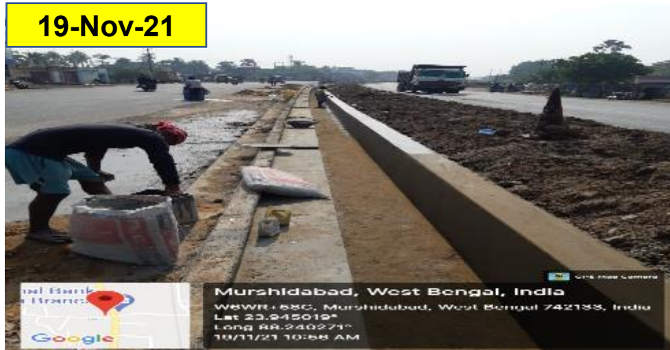
Km 180+365 median drain WIP
