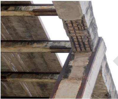
Figure 3.15: Pipe Rack Damages
