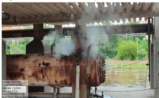
Figure 3.2: Plant 2 Primary Reformer Leak
