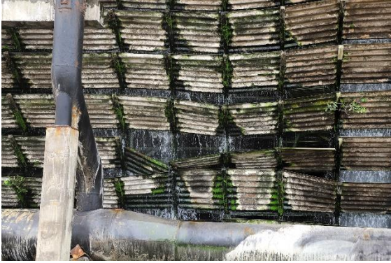
Figure 3.13: Cooling Tower Damages
