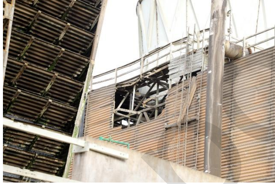
Figure 3.14: Cooling Tower damages
