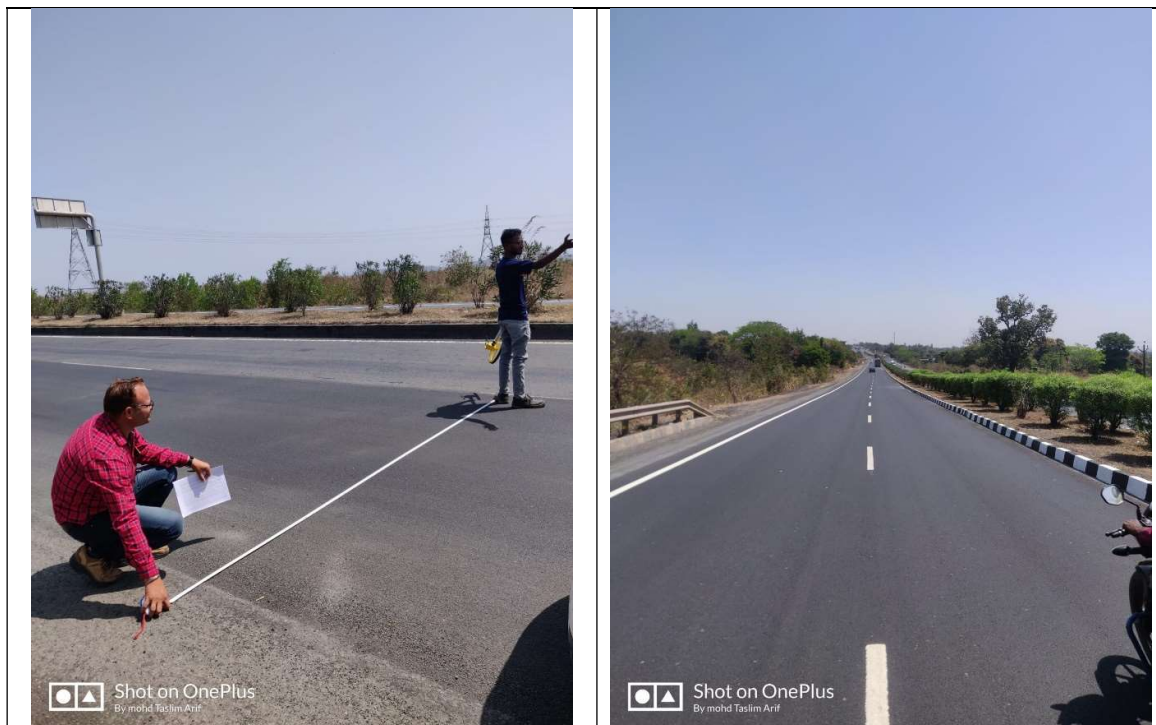
BC work after milling were completed also the road marking
