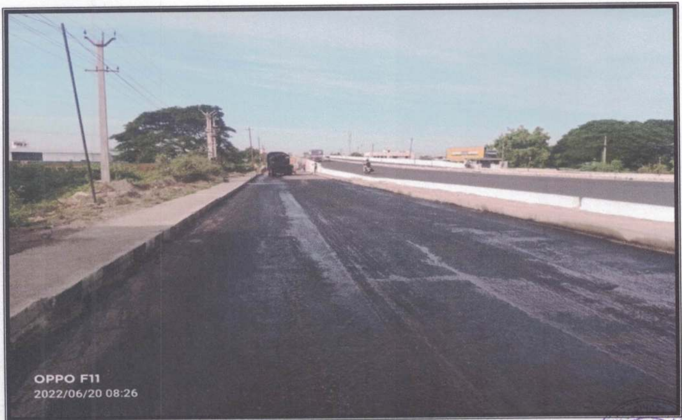
CONSTRUCTION OF VUP BLACK SOPT AT KM297+000- APPLYING OF TACK COAT FOR BC LAYING ON SERVICE ROAD
