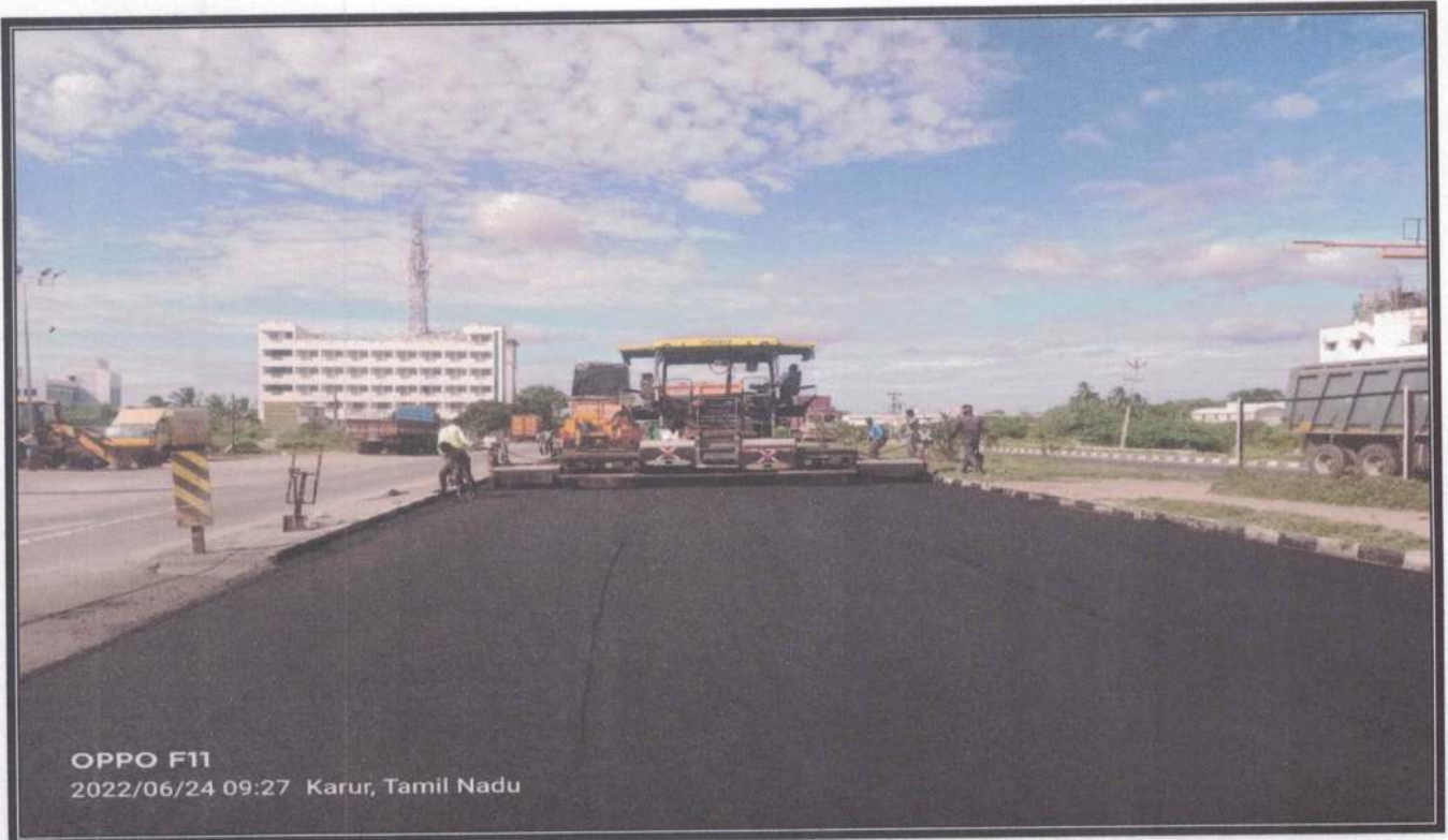
CONSTRUCTION OF VUP BLACK SOPT AT KM297+000- BITIMINOUS CONCRETE LAYING WORK
