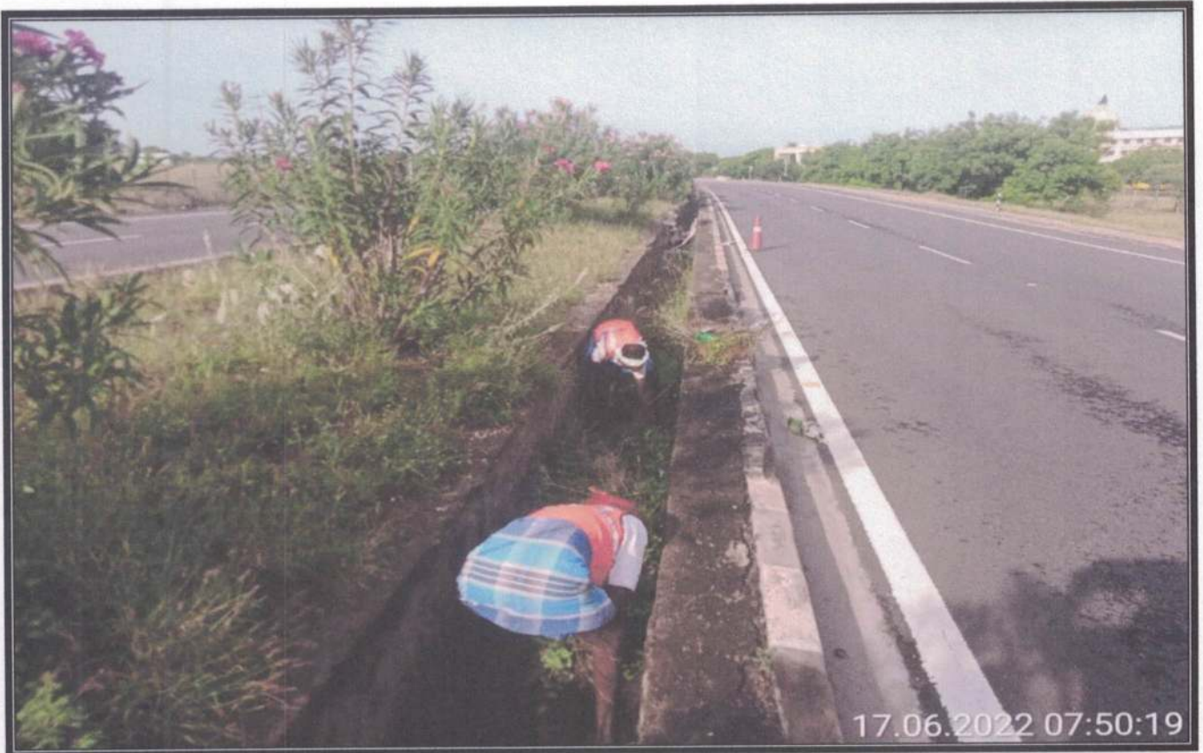
MEDIAN DRAINAGE CLEANING WORK
