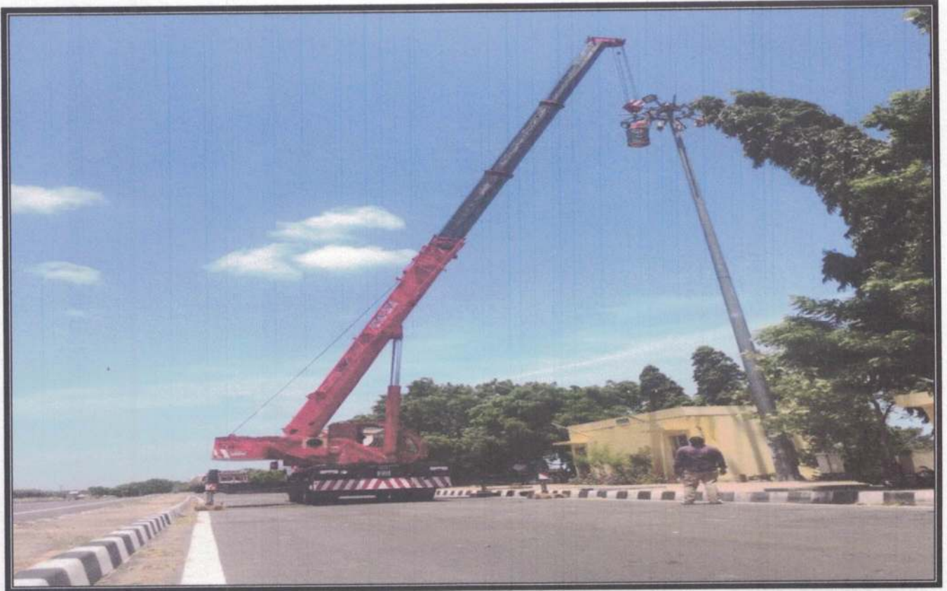
TRUCK LAYBYE AT KM:326+000-RHS HIGHMAST LIGHT REPAIRING WORK
