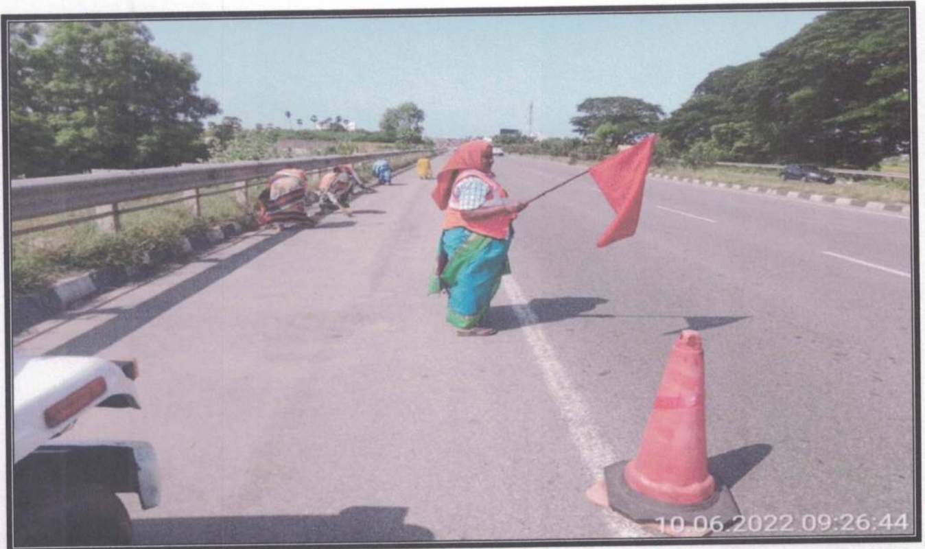
ROUTINE MAINTENANCE WORK
