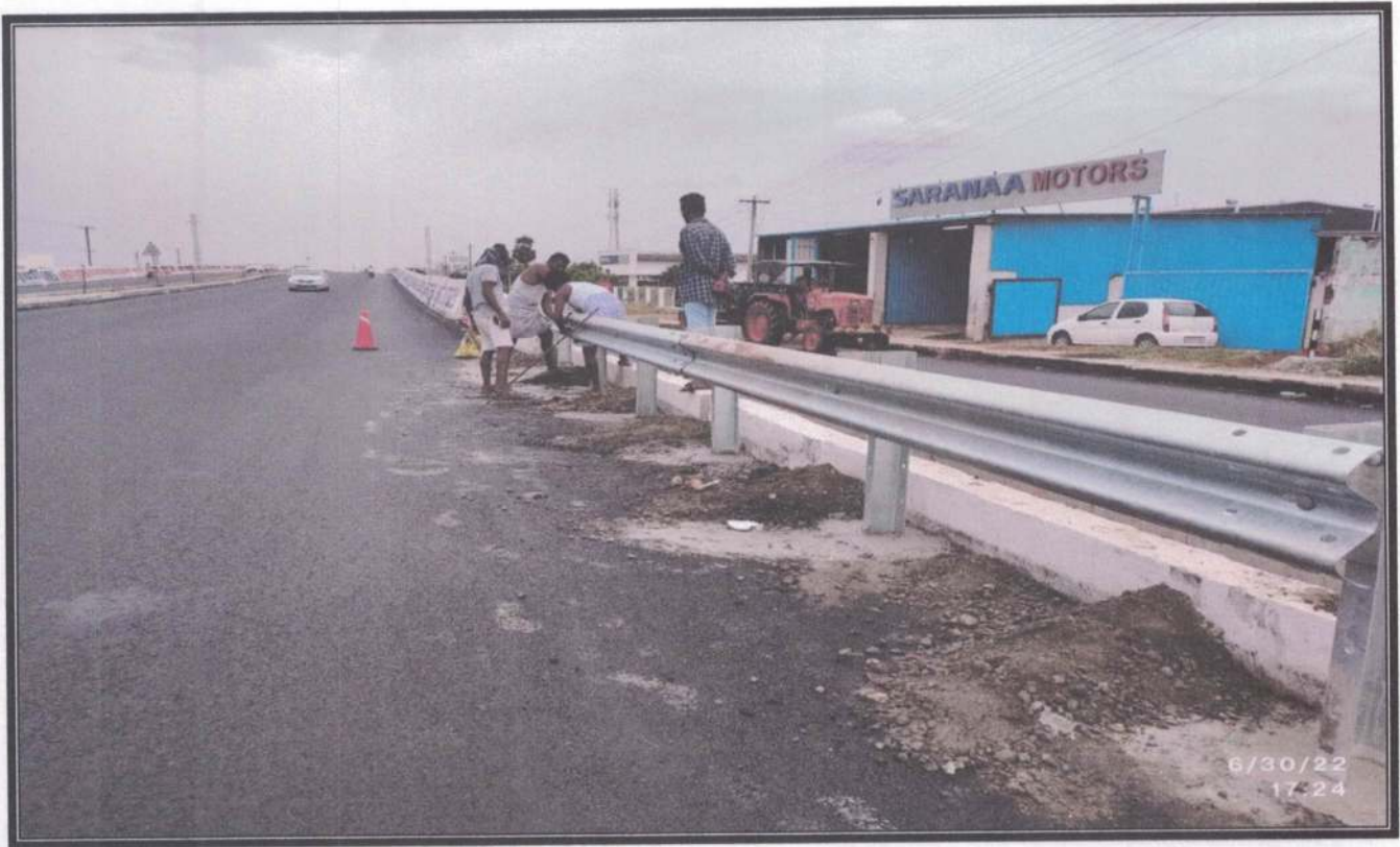
INSTALLATION OF METAL BEAM CRASH BARRIER ON CONSTRUCTION OF VUP BLACK SOFT AT KM293+000-END OF APPROACHES
