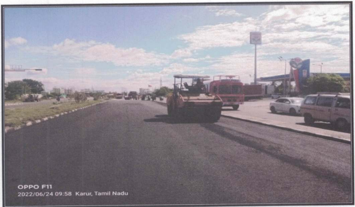
CONSTRUCTION OF VUP BLACK SOPT AT KM297+000- BITIMINOUS CONCRETE COMPACTION WORK
