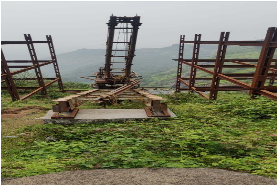
LAUNCHING GIRDER AT UPPER STATION
