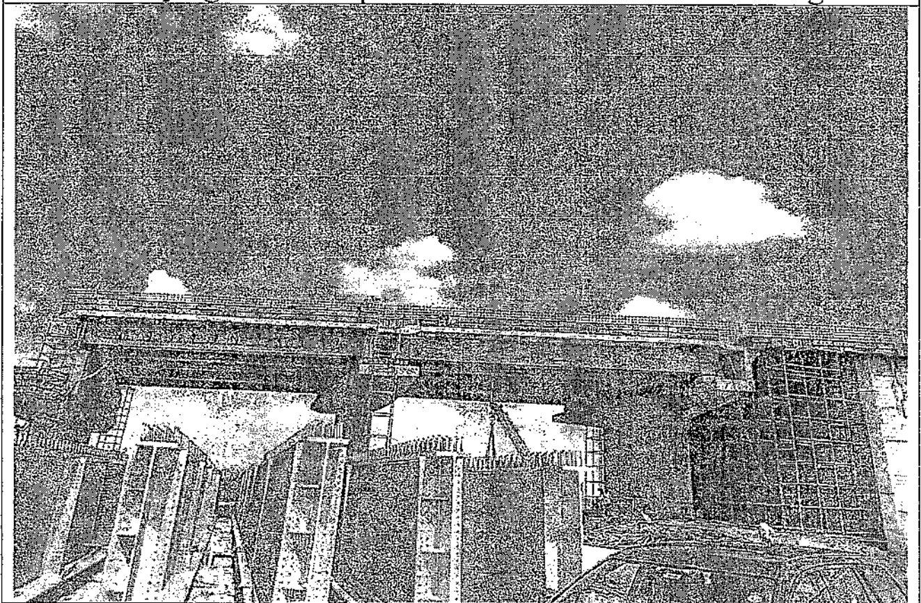
Assembling work of Plate girder is completed ready for launching
