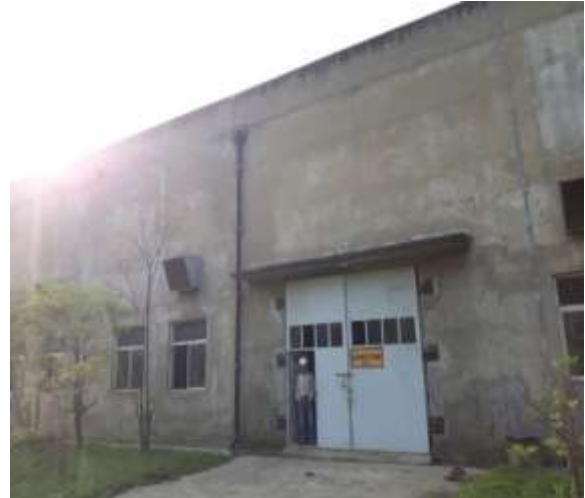
Ash water pump house
