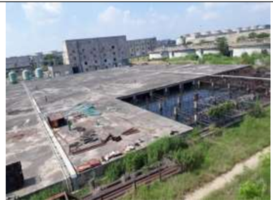
CWST storage Tank
