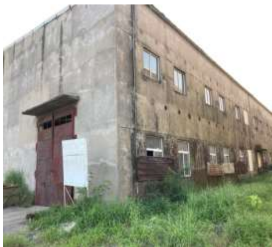
Closed storage shed
