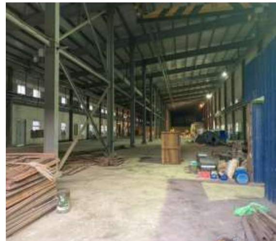
Internal view of closed storage shed
