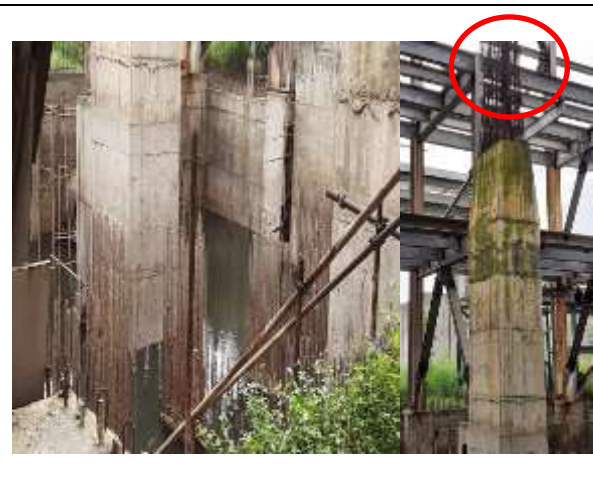
TG deck foundation is incomplete and some of the portion is submerged in water. Rebars of the RCC structure are also in corroded condition. Needs immediate attention to protect damage to RCC structure.
