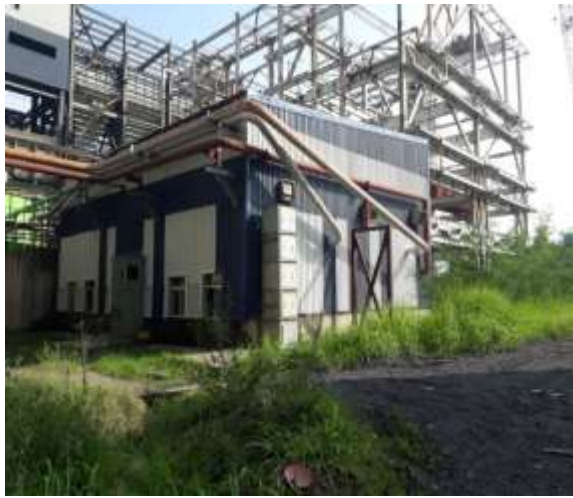
Ash Slurry pump house
