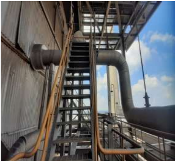
Condition of cladding and piping insulation found in good condition
