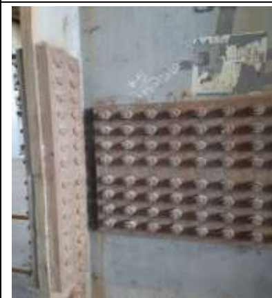
Condition of TG structure- General corrosion observed and all such location needs to be painted.
