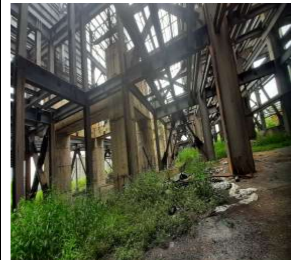
Foundation of Mill area. Foundation studs are found in good condition, however certain studs needs to be protected to prevent damage
