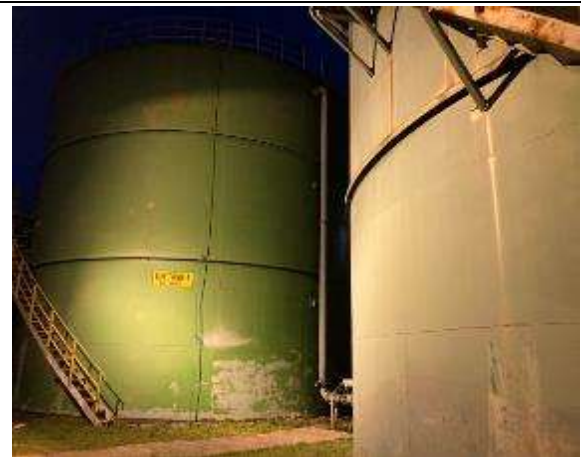
4X1600M3 Capacity DM Tanks
