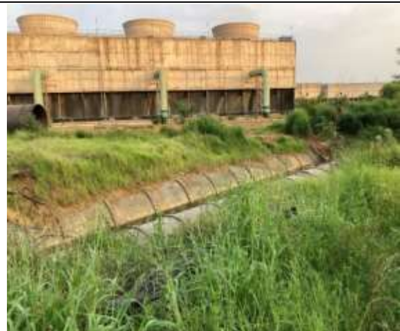
Exposed CW UG pipelines
