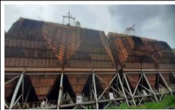
Construction of ESP and duct under progress
