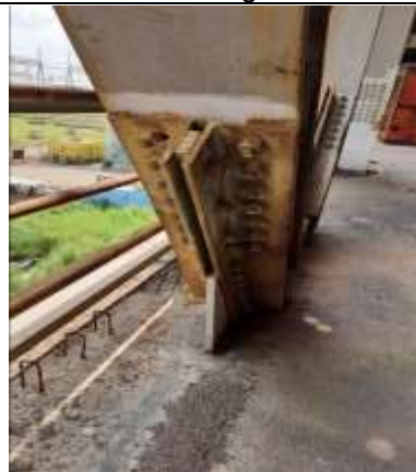
Condition of TG structure- General corrosion observed and all such location needs to be painted.
