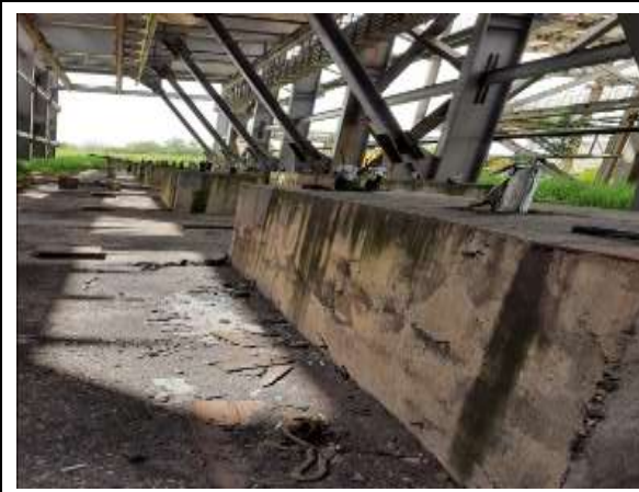
Foundation of Mill area. Foundation studs are found in good condition, however certain studs needs to be protected to prevent damage
