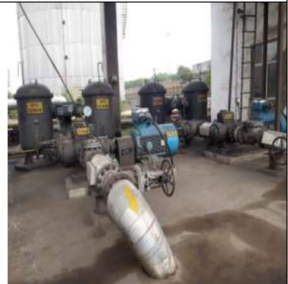
HFO pump and piping
