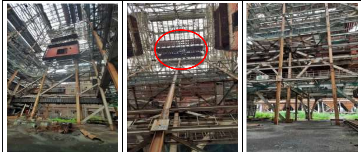
Construction of pressure parts under progress. Pressure parts are marked in photo
