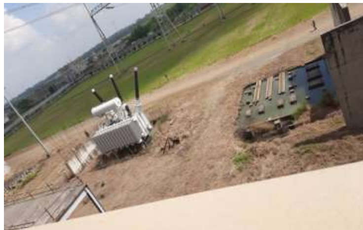
ST placed on foundation
