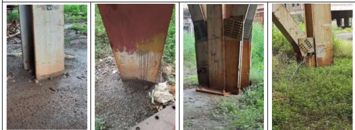
Condition of Boiler structure. Some of the structure is embedded in soil/vegetation. Needs to be attended to prevent damage due to corrosion.
