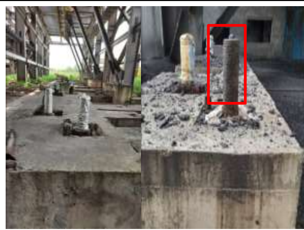
Foundation of Mill area. Foundation studs are found in good condition, however certain studs needs to be protected to prevent damage
