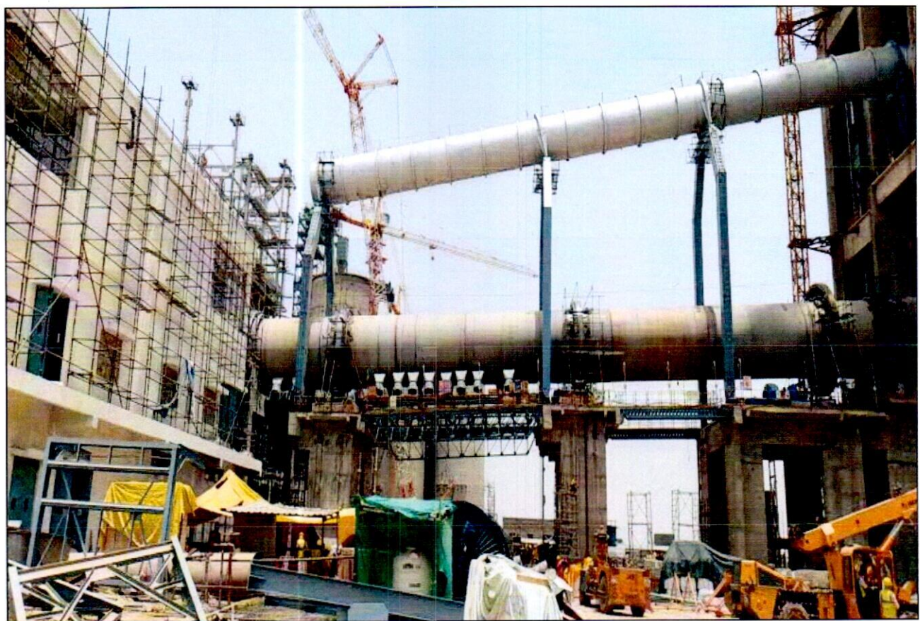
Klin, Kiln Piers & TA Duct and support structure
