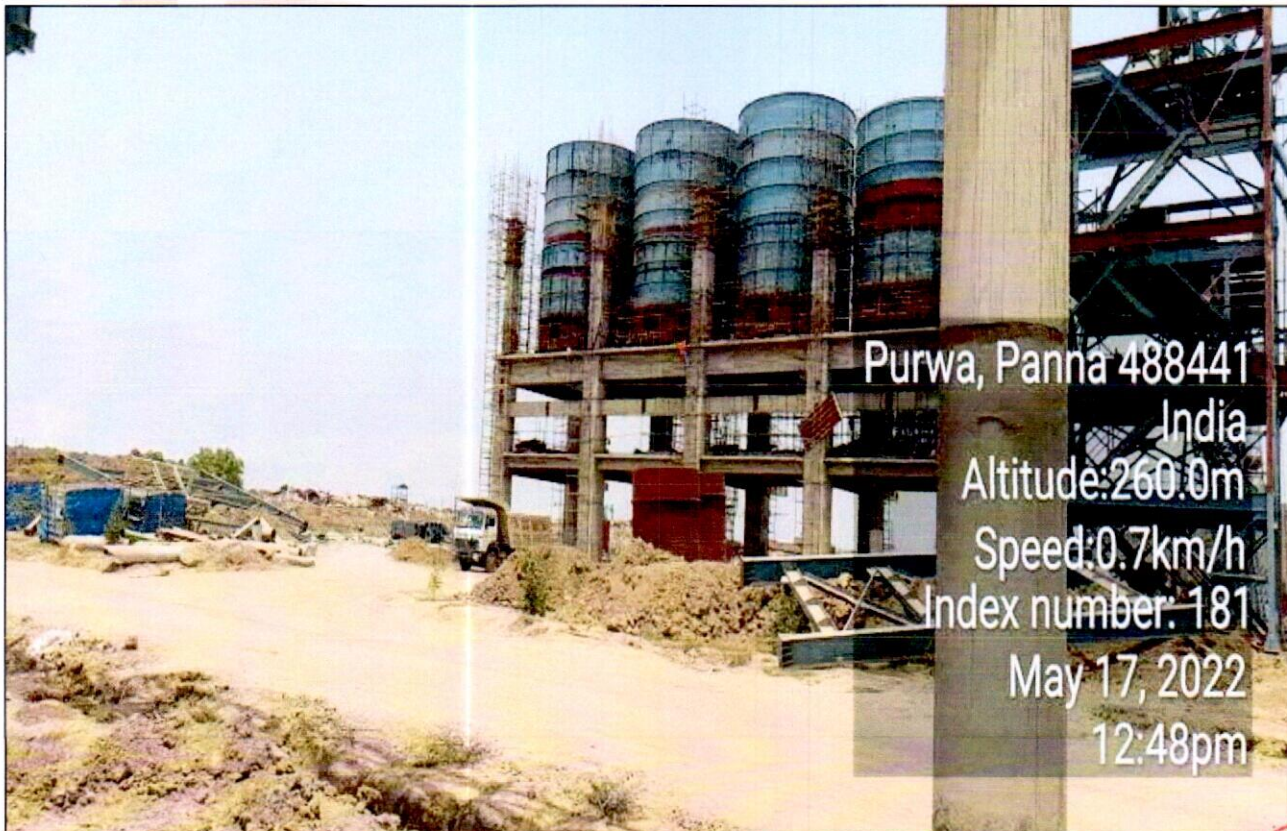
Clinker Load out Hoppers
