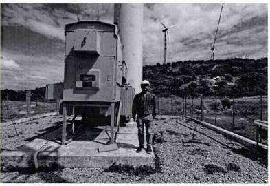
The power generated by wind mill transmitted by underground Cables to this generator/ convertor in picture above which converts 690 V to 33 kV for transmission.
