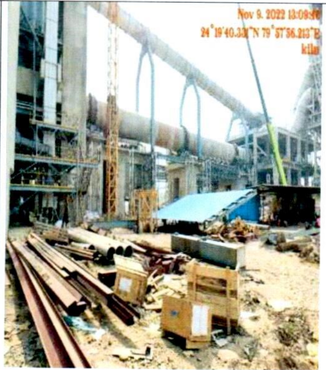
KILN AND TA DUCTS
