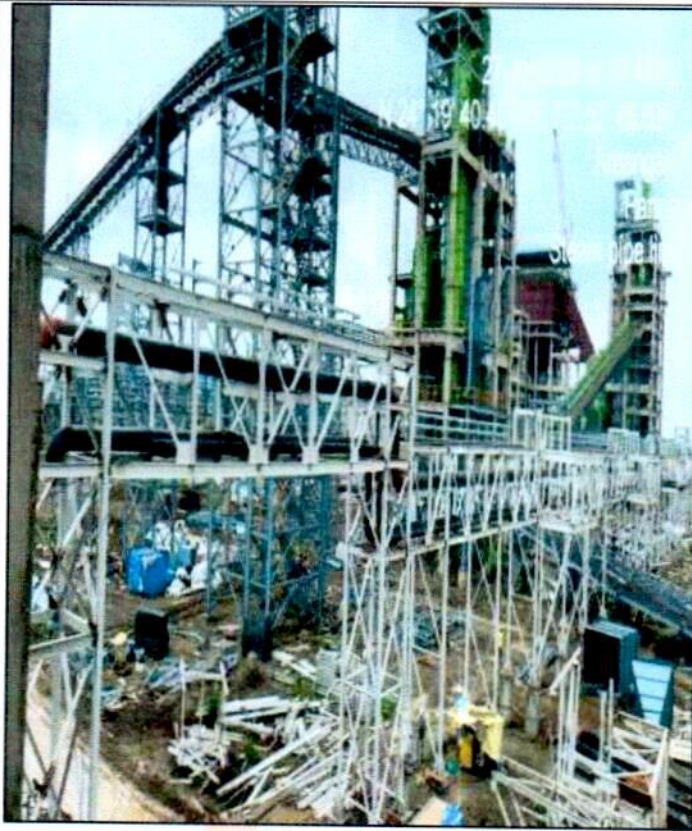
HOT AIR PIPELINE AND CABLE GALLERIES
