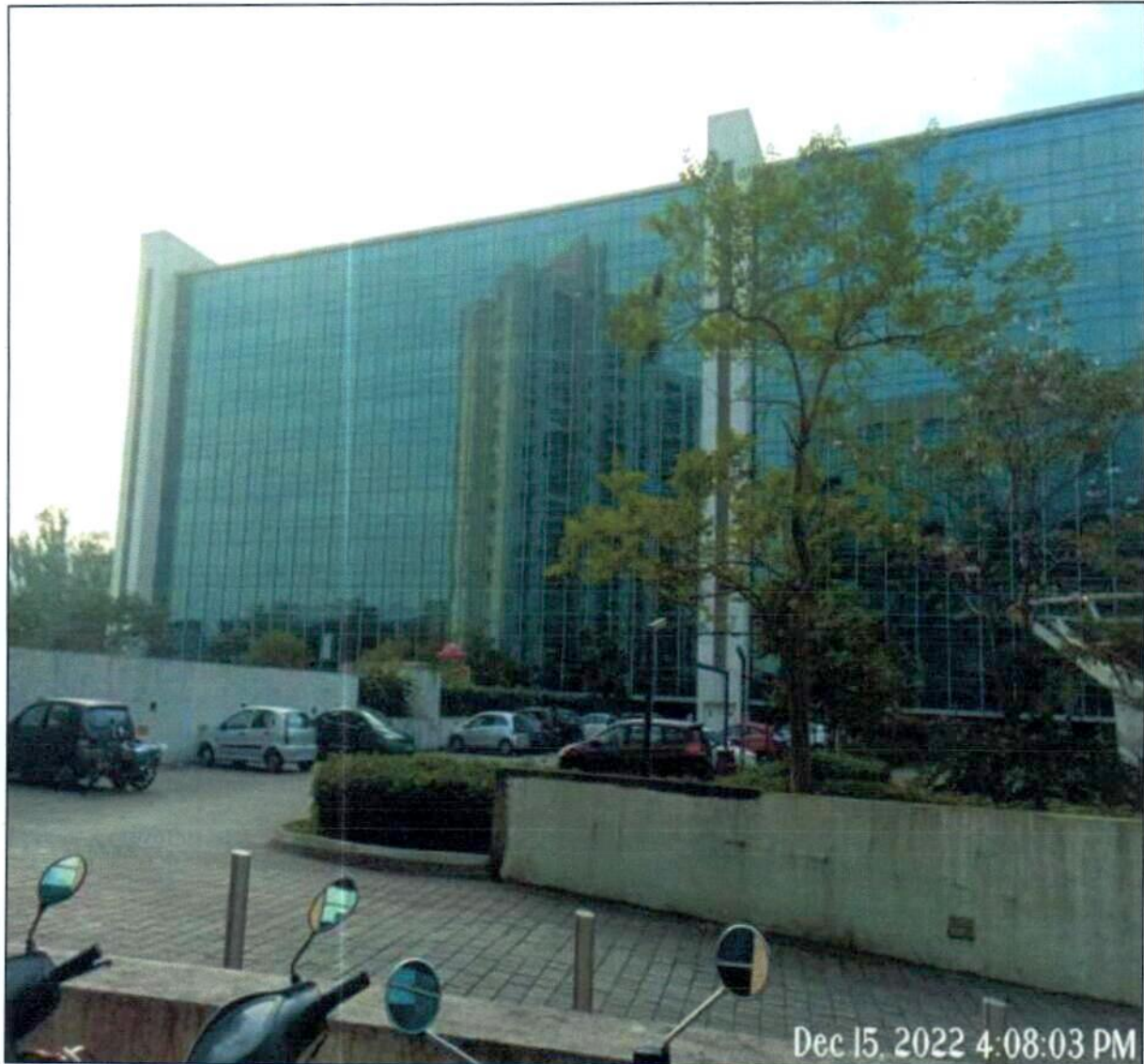
LODHA SUPREMUS-II, PHASE-II, UNIT NO.617, 6TH FLOOR, PLOT NO. F-4 & F-4/1 ROAD NO.22, WAGLE ESTATE (W), THANE-400604
