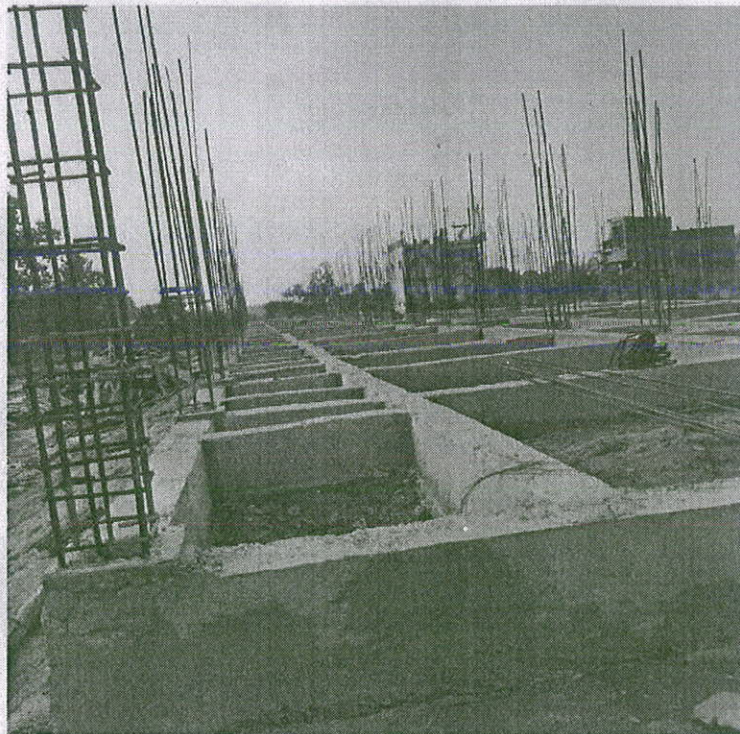
VIEW OF PLINTH BEAMS
