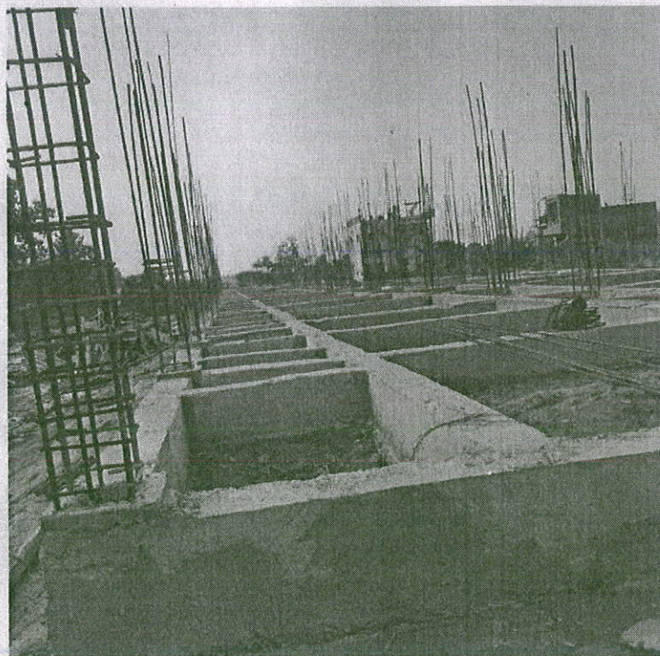
VIEW OF PLINTH BEAMS
