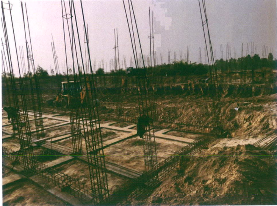
VIEW OF PLINTH BEAM REINFORCEMENT
