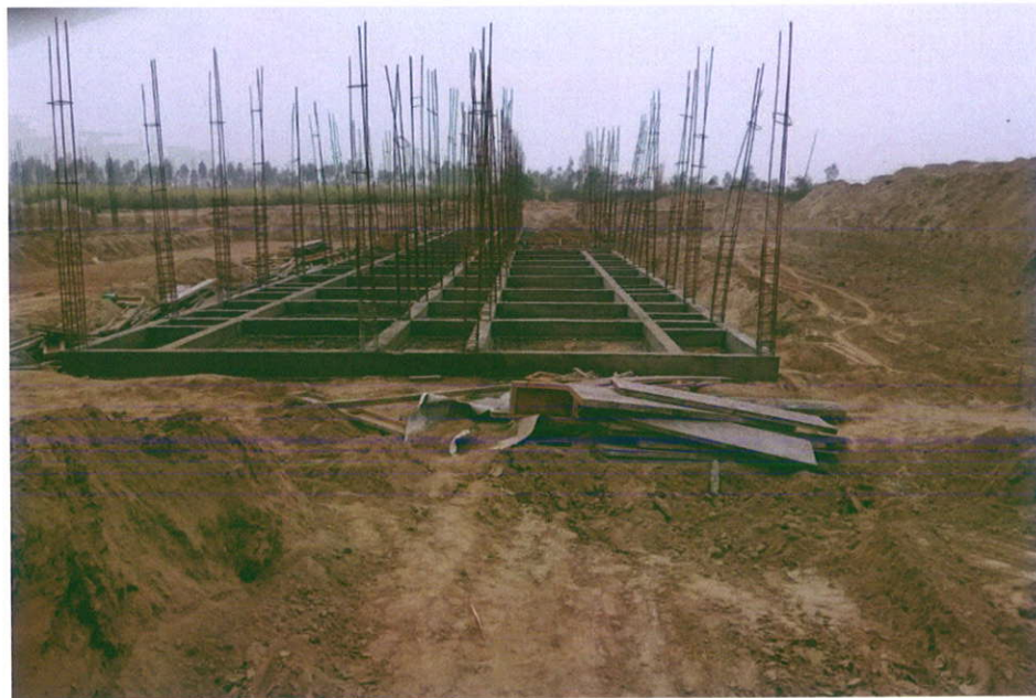
VIEW OF PLINTH BEAMS
