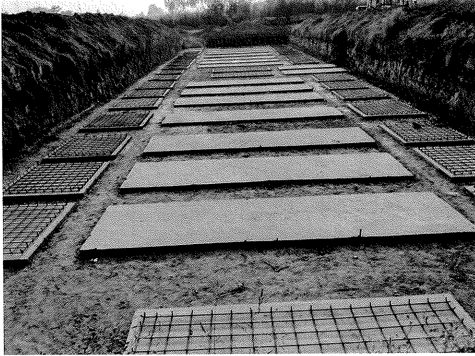
VIEW OF PCC AND FOUNDATION REINFORCEMENT
