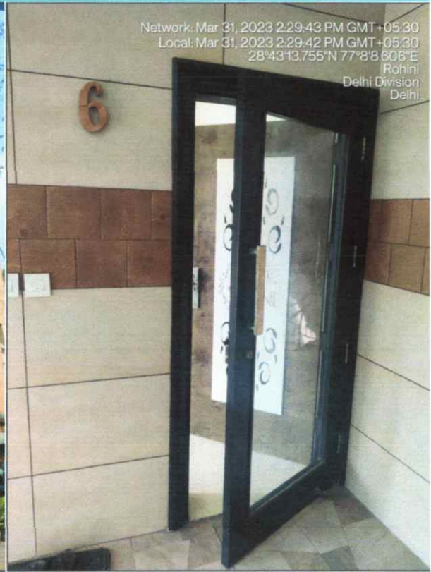
Flat No.06 Entrance Door
