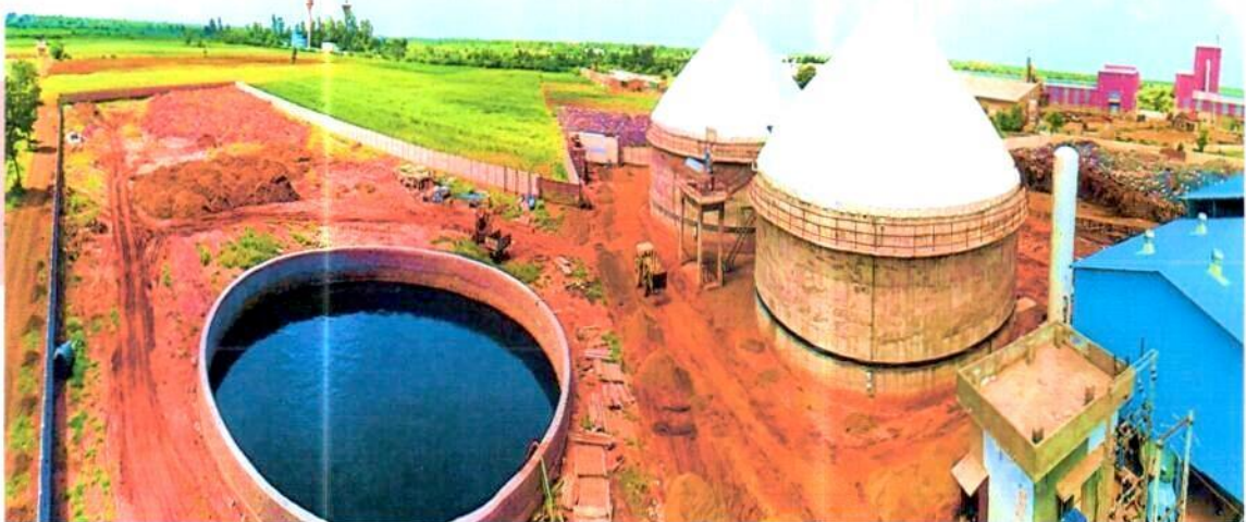
CSTR Technology based Anaerobic Digester
