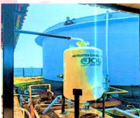
H2S Removal -Biogas cleaning
