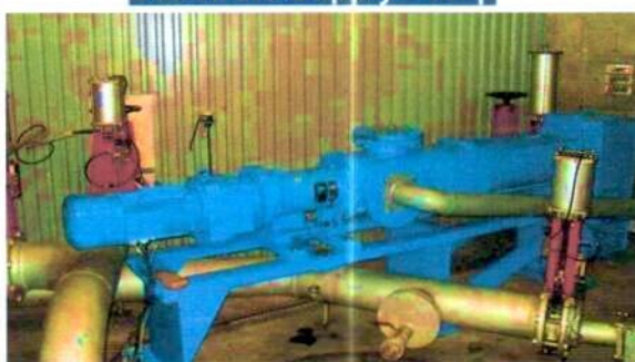
Substrate Supply Pump
