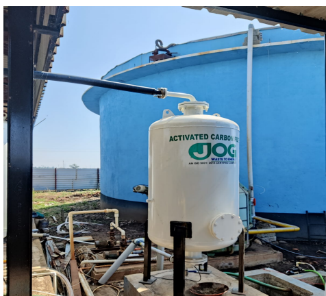
H 2 S Removal -Biogas cleaning system
