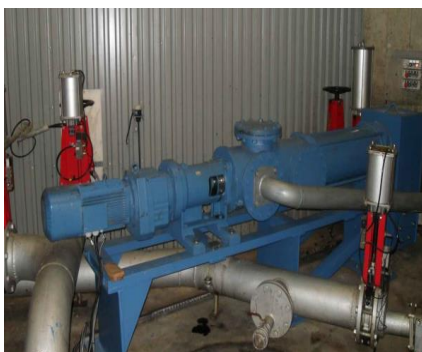
Substrate Supply Pump
