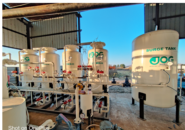
Moisture & Co 2 Removal -Biogas
