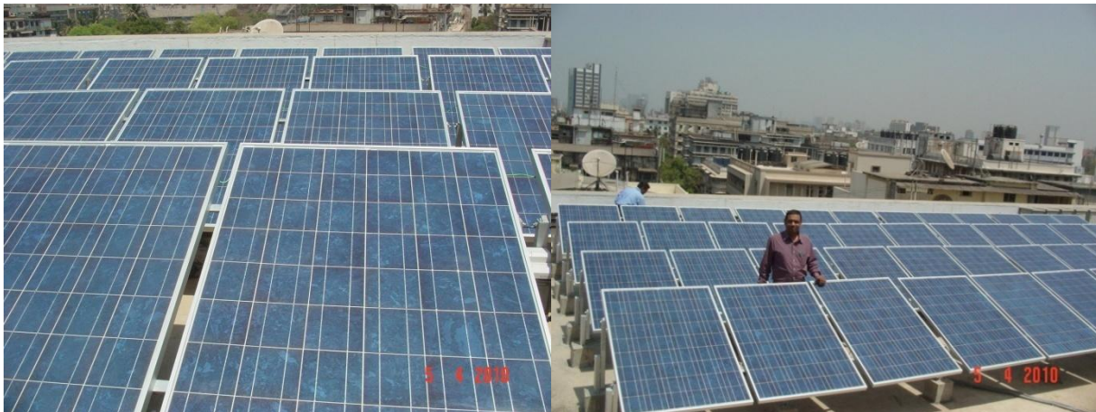
Grid Tied 10KW Crystalline Solar PV installed at Mumbai.
