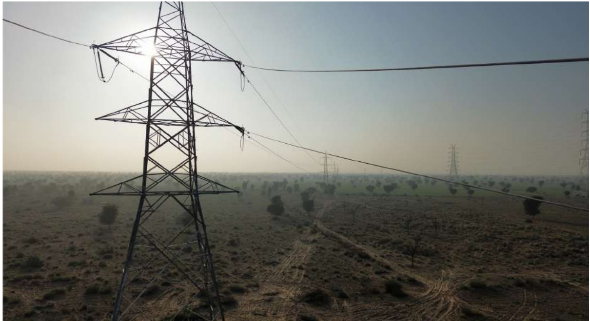
Power evacuated through a 220 kV Switchyard and 11 km 220kV transmission line with HTLS conductor
