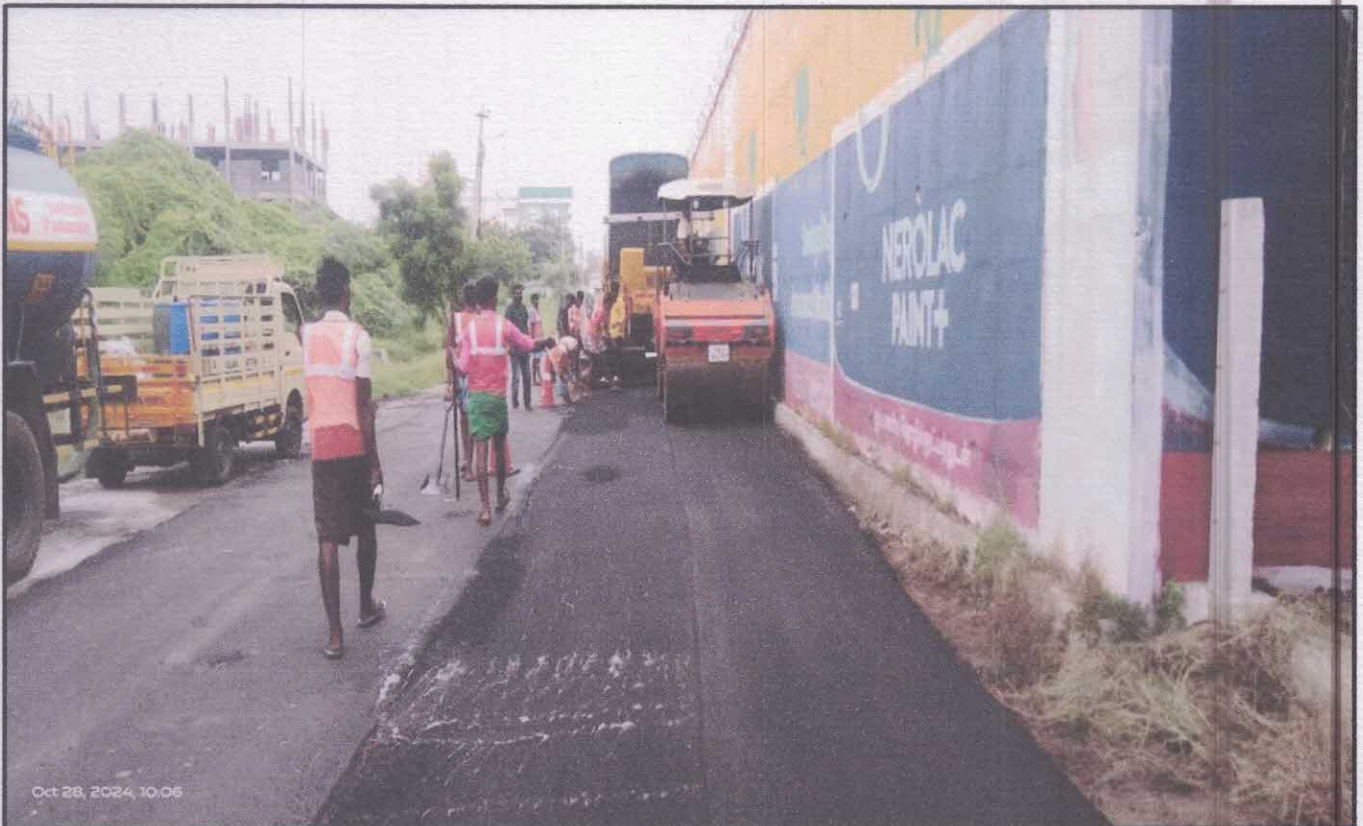
Karur Bypass Service road BC relaying work
