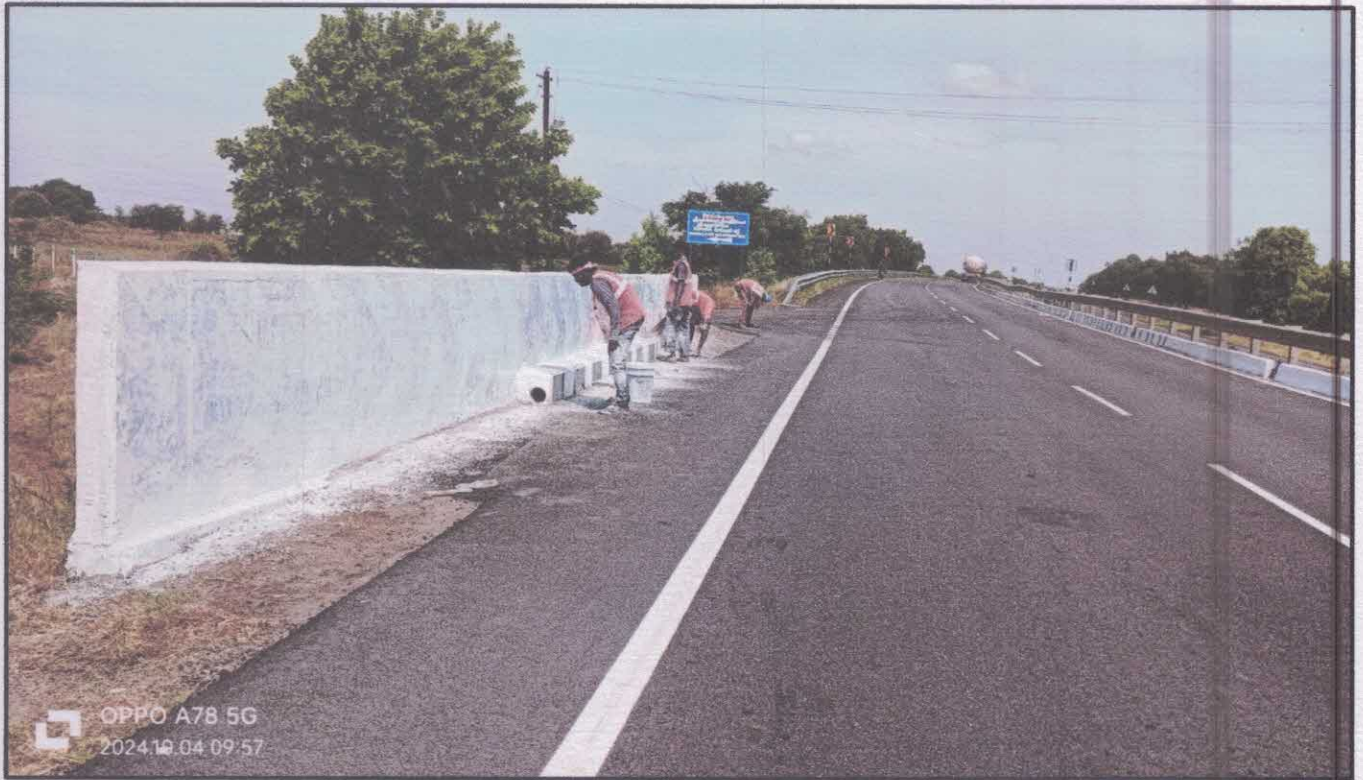
Crash barrier illegal adverdisenment hoarding removal & re painting Work
