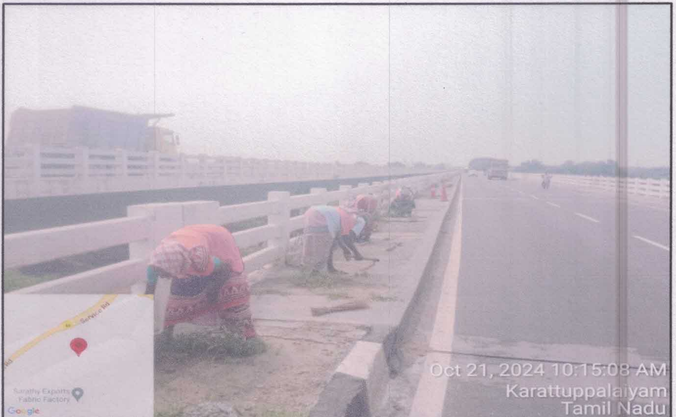
Major Bridge foot path portion unwanted weeds cleaning work
