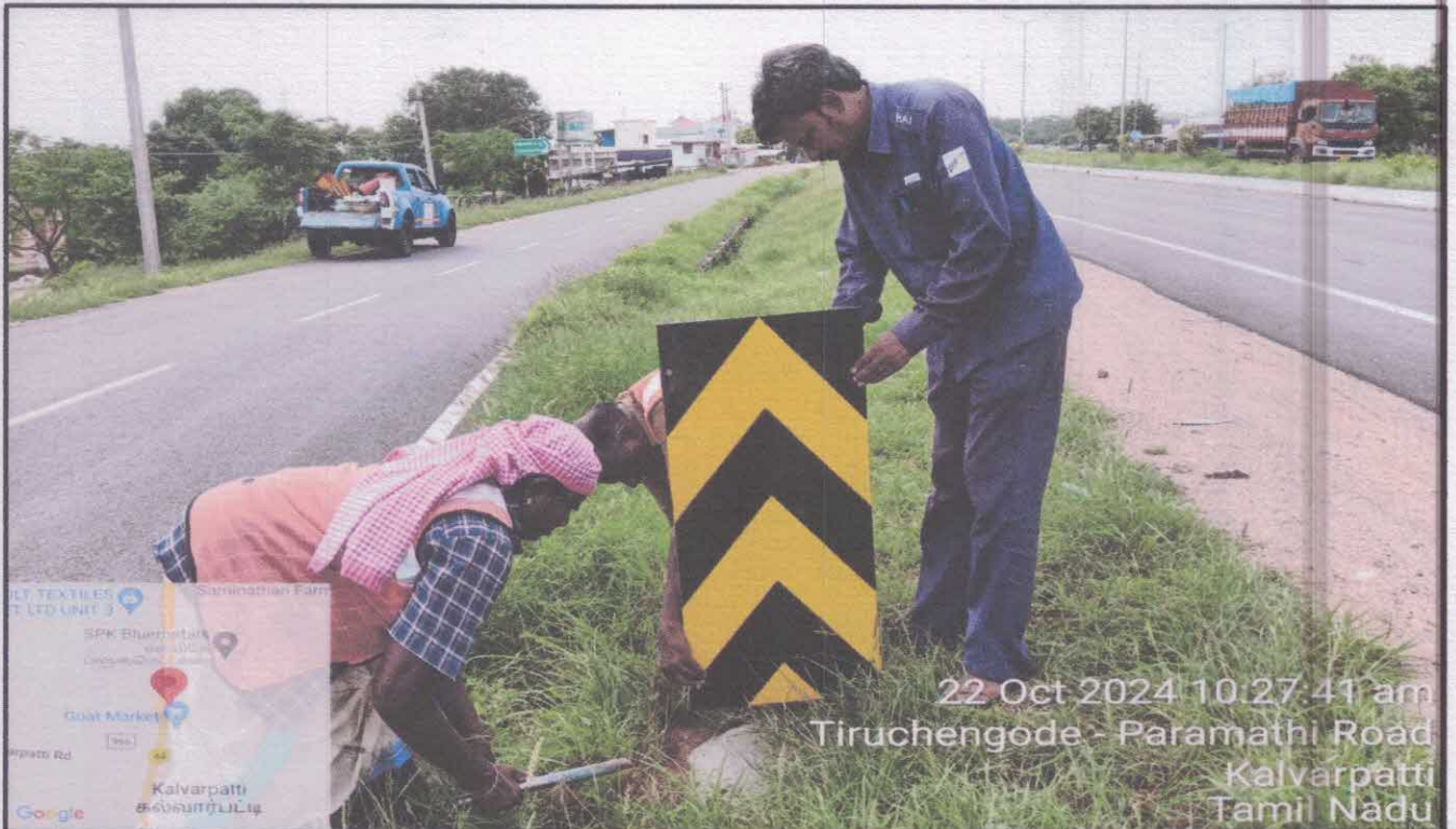
Installation of two way hazard marker sign
