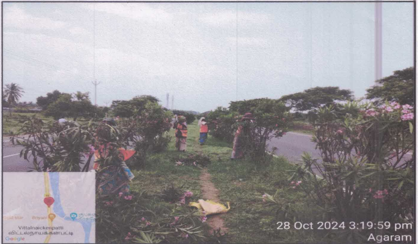
Median Plantation Trimming Work
