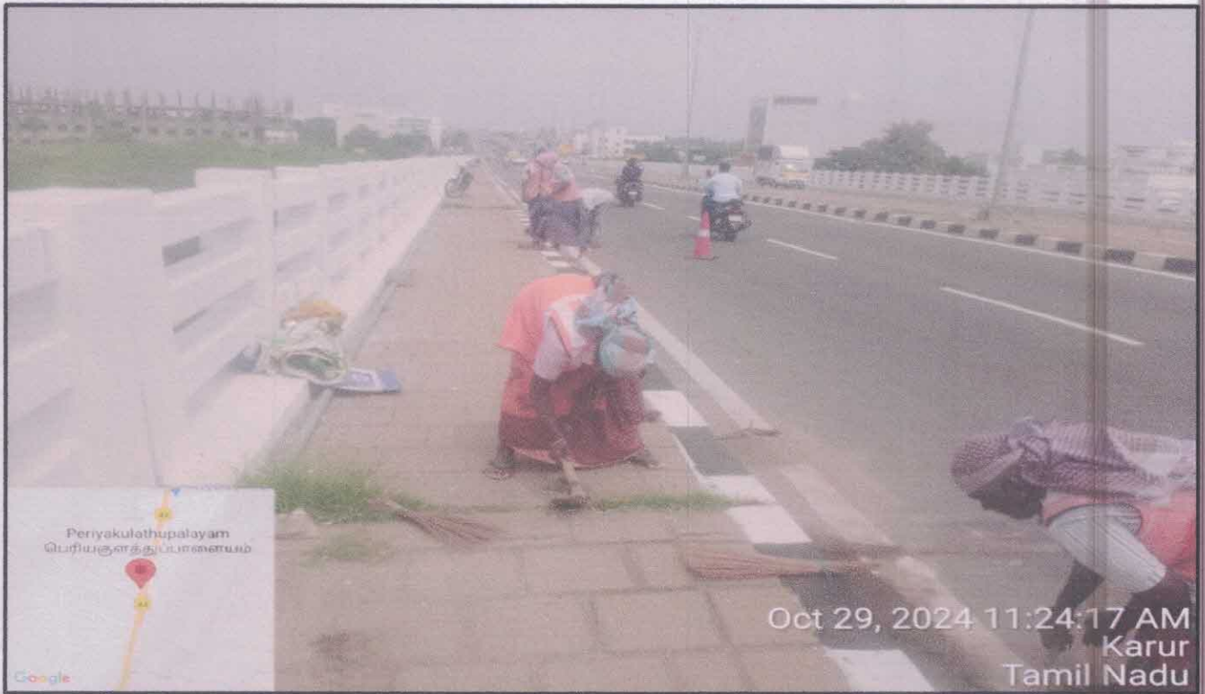
Routine Maintenance Work
