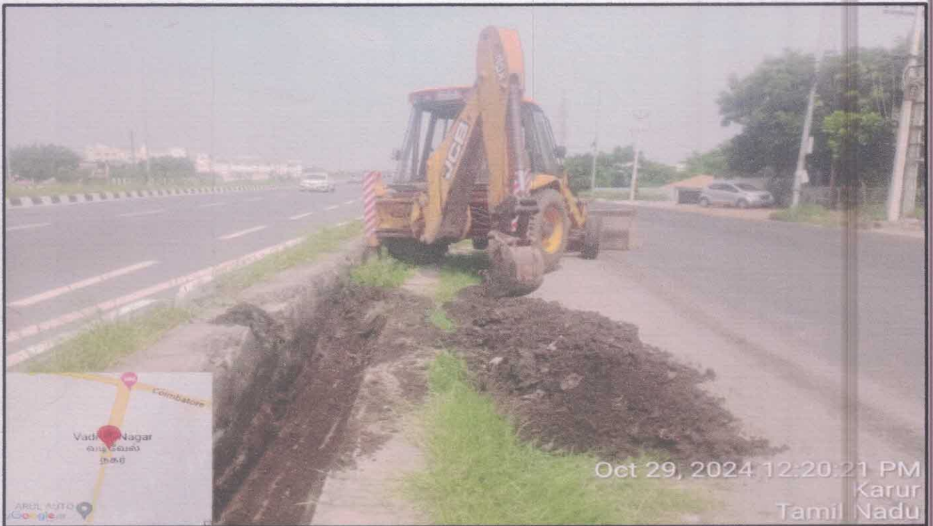
Chocked drain cleaning work
