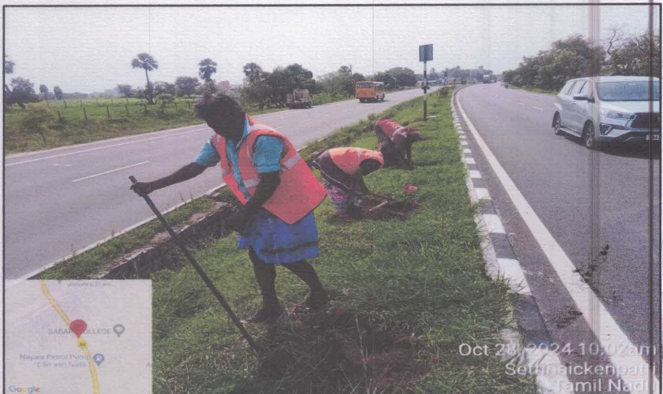
Pitting work for Median plantation
