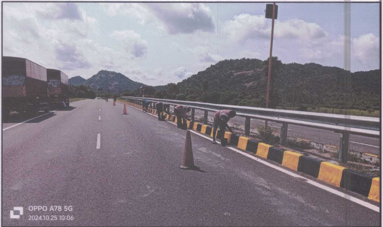
Kerb Painting Work
