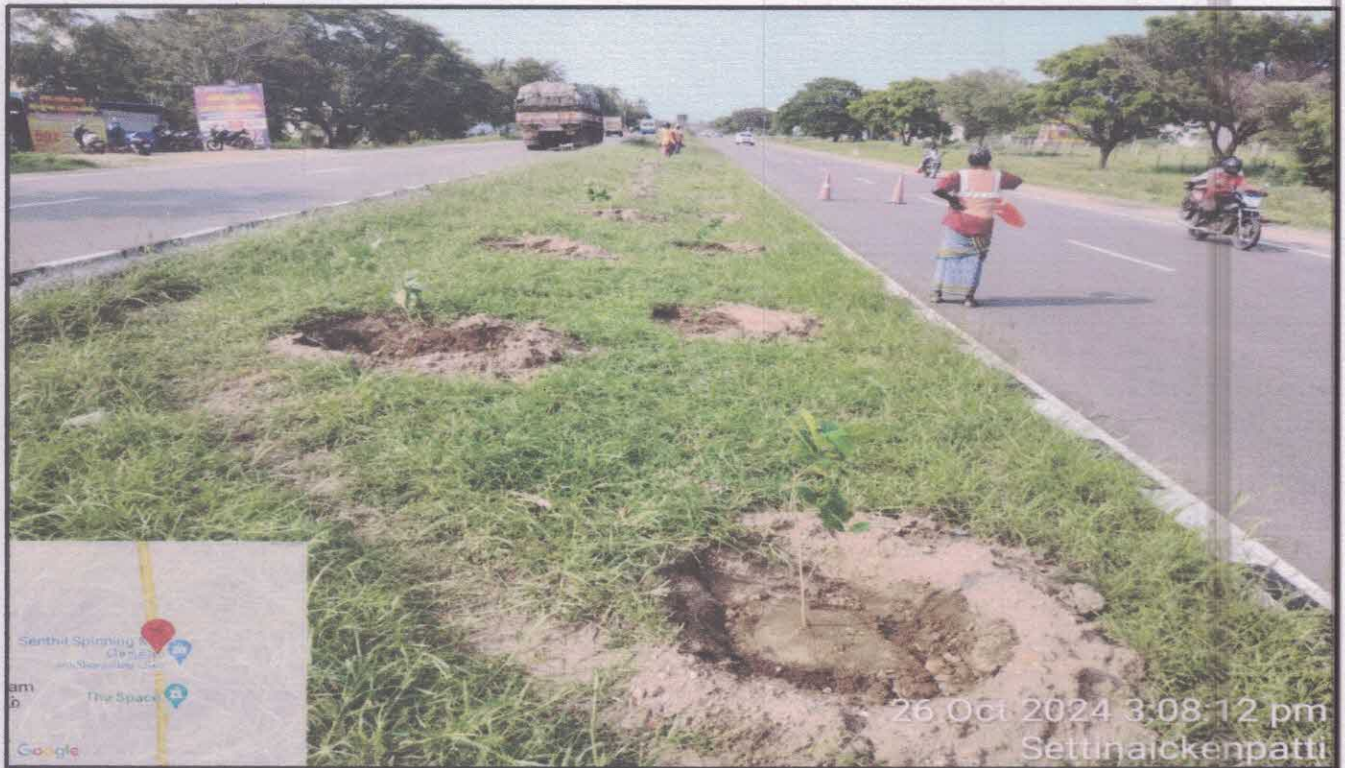
Median plantation planting work
