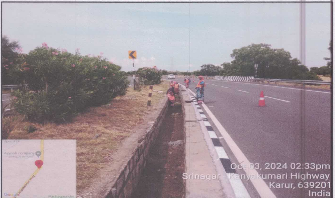
Median Drain Cleaning
